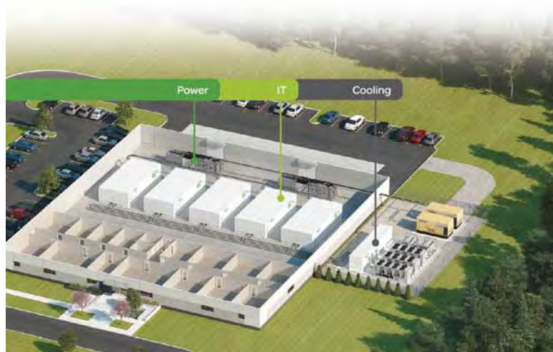
Prefabricated data centre modules.
